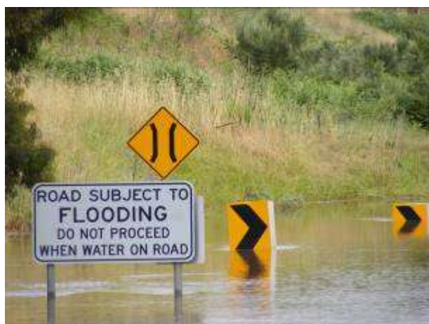
Oaks Estate Rd Crossing, at the height of the December flood. (John Bruggeman)
