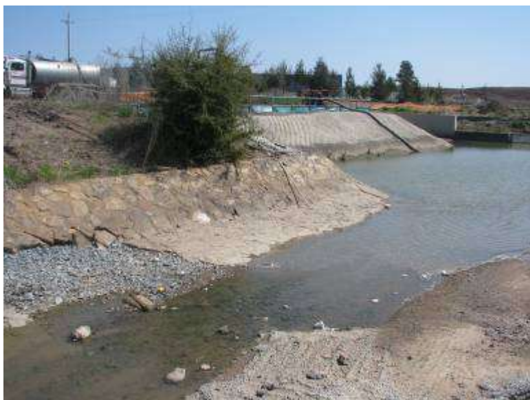
Weston Creek below Cotter Rd, as a construction site.
